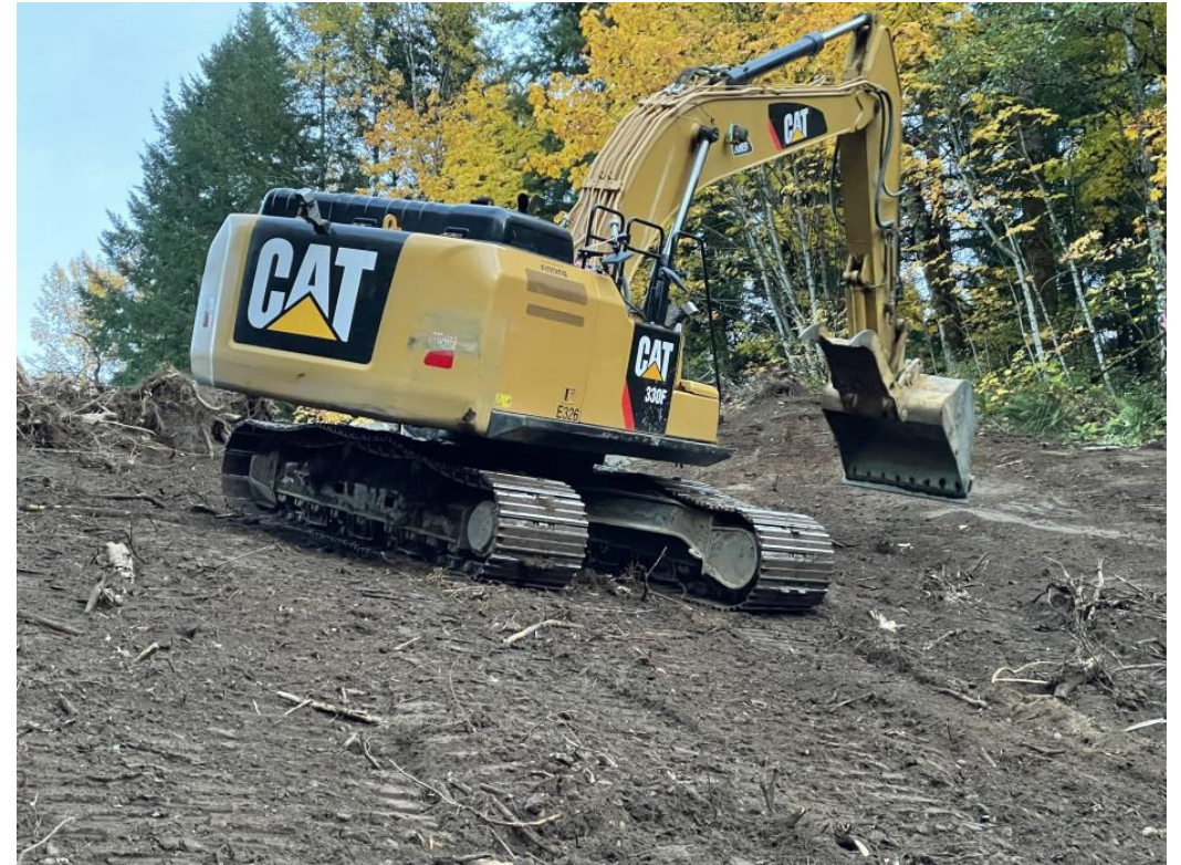
Track packing of replaced topsoil.
