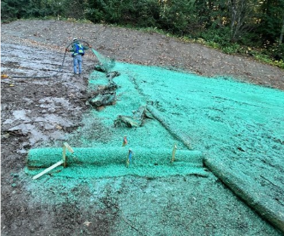
Hydroseeding and ESC measures in place.
